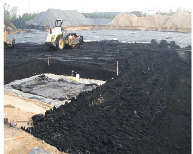
Figure 2: Disposal of Waste Foundry Sand
